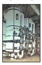
There is a great inherent advantage in using columns for sorption – they can come in a of range sizes. From very small "cannisters" (even portable) to the largest size as seen in the picture. For flow-rates, high columns can be multiplied into sets of many (paralell) unlimited for process scale-up.
